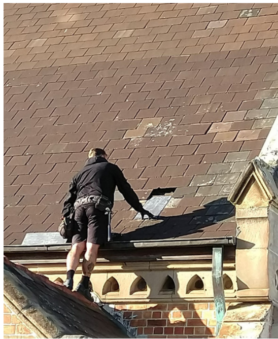
REPAIRING LOOSE TILES ON ROOF
